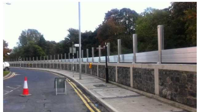
Photo 2: Flood wall consisting of permanent wall, and demountable wall adjacent to a sidewalk/road.
