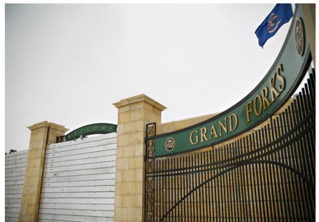
Photo 8: Flood wall installation with demountable wall in some sections.
