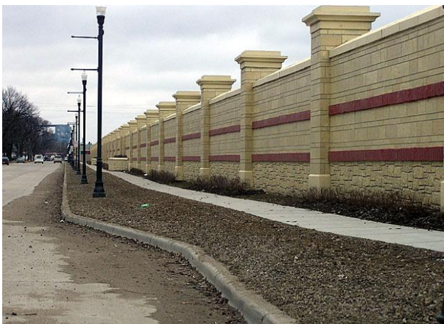
Photo 7: Permanent flood wall installation.
