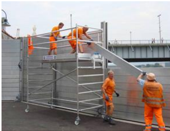
Photo 6: Flood wall installation.
