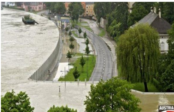
Photo 1: Flood barrier by IBS.
